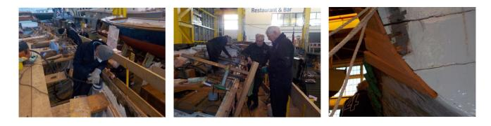
up the top of the port riser, next on previous page Jeremy, Mike F and Roz R are working on one of the last 'long' planks using a shore and a 'big man's' clamp to pull the top into shape. Far right is one of our earlier attempts to sort out the final section of planking adjacent to the transom. All to no avail, so back to the drawing board on this one.
