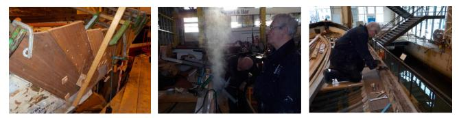
Above left a general shot looking aft at some of the planks in place. Over right in the middles two Mikes are steaming a stubborn plank or are they really making a cup of tea. The time had finally come to make a start on the starboard inwale and gunwale capping and above right Steve F has been cutting off the gunwale capping so that we could assess the inwale. It turned out that it was like the curate's egg, Good in parts. Below left Jeremy C is way down aft tucked up against
