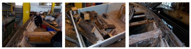
the transom removing some of the rotten inwale. Above middle shows some of the gunwale capping that had been removed I thinks that in general it proves the point of cutting it out. Above far right you can see some of the poor parts of the curate's egg, or in this case the dodgy inwale which will be cut out and replaced.
