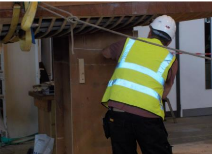
are fitting the main lifting straps. Having taken the weight on the crane Tiger is underneath with his sabre saw cutting away at the building blocks and finally above right he cuts through the stem leaving the boat to 'float away' up to the ceiling.
