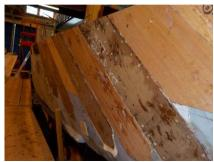
most of the clamps removed and some of the copper nailing complete along with an initial degree of fairing. Top of the next page left shows Hamo and Roz working on the copper nailing and screwing some of the boards in place. Middle is Roz at an impossible angle in the boat riveting Hamo's nails and far right two fairly new starters Micky and Sam clearing the decks a little before getting stuck into the rotten timber in the starboard inwale.
