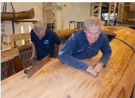
sanding down the hull planking overall. Below left John is making lots of shavings along with Igor as they are doing some of the final fettling to any high spots in the plank seams. Below middle Ian P, John and Mike S are cleaning up the corners in the cockpit ready to start planning the coaming.
