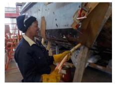
bring the beast into submission steaming it, bending it, shoring it, wedging it, bolting it and finally nailing it into Sounds place. good doesn't it, well it would have been if the beast had been lying close to the inner planks all round
