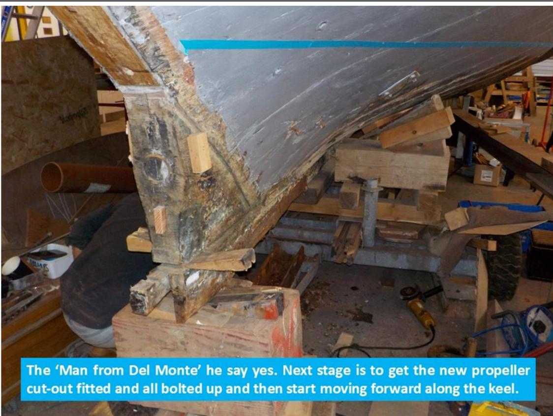
The 'Man from Del Monte' he say yes. Next stage is to get the new propeller cut-out fitted and all bolted up and then start moving forward along the keel.
