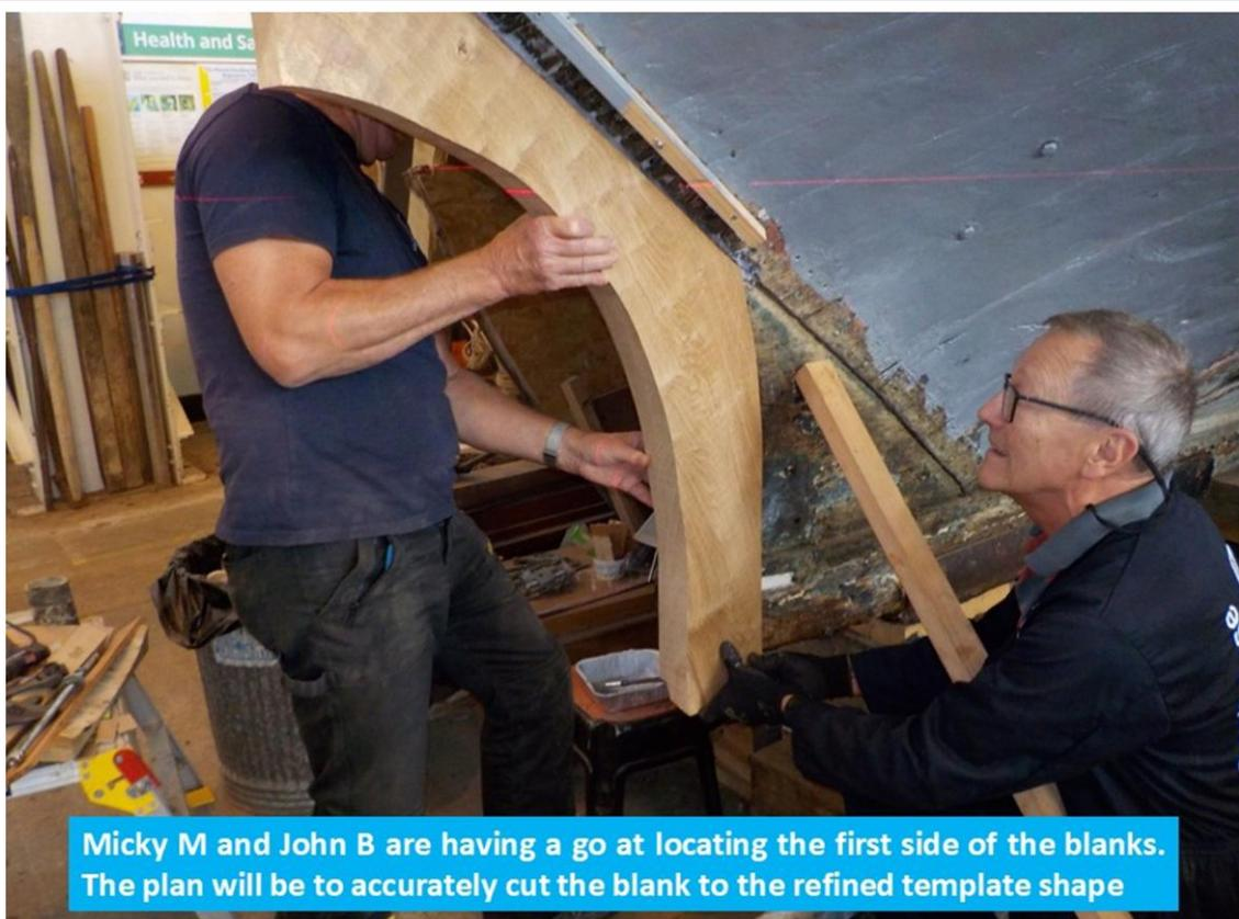
Micky M and John B are having a go at locating the first side of the blanks. The plan will be to accurately cut the blank to the refined template shape
