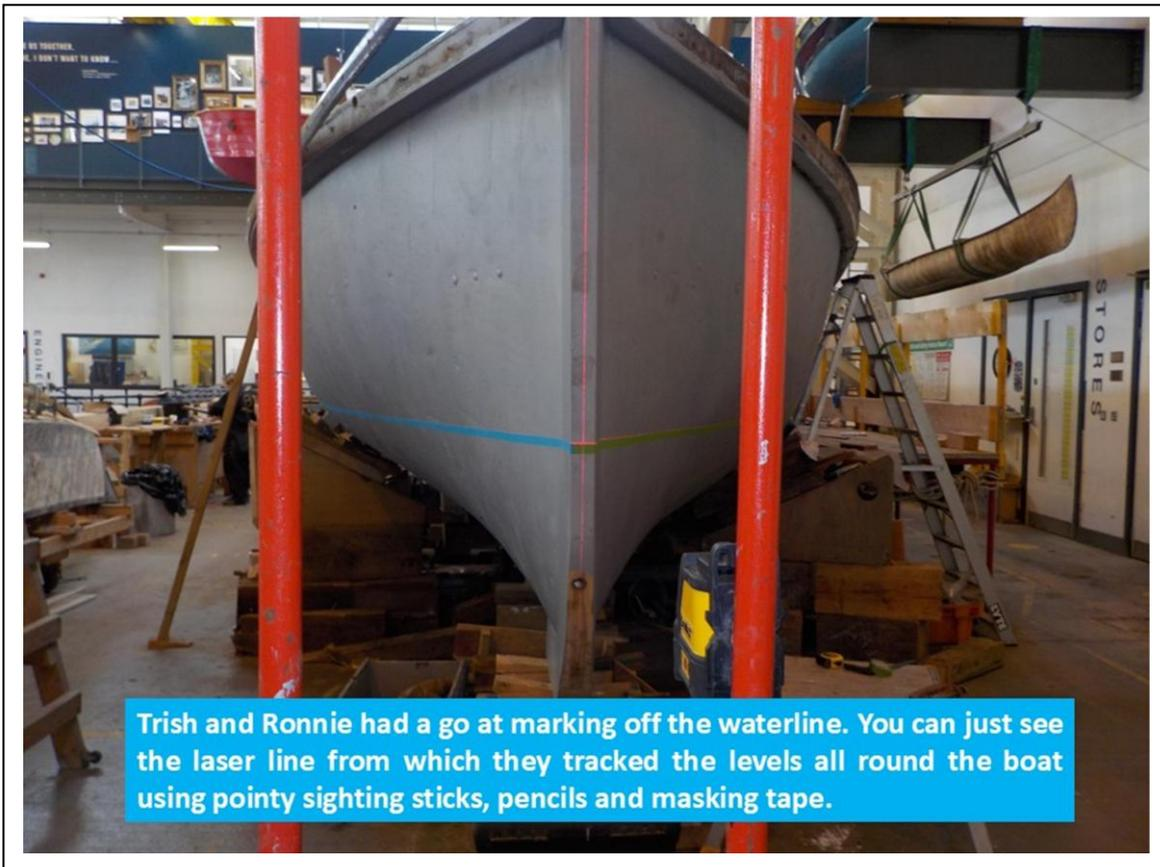
Trish and Ronnie had a go at marking off the waterline. You can just see the laser line from which they tracked the levels all round the boat using pointy sighting sticks, pencils and masking tape.
