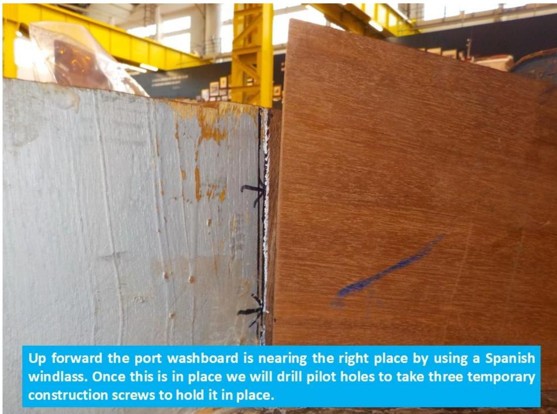
Up forward the port washboard is nearing the right place by using a Spanish windlass. Once this is in place we will drill pilot holes to take three temporary construction screws to hold it in place.
