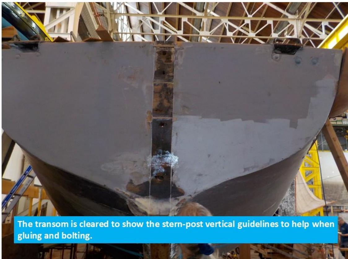
The transom is cleared to show the stern-post vertical guidelines to help when gluing and bolting.
