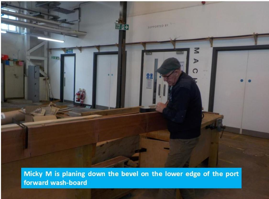
Micky M is planing down the bevel on the lower edge of the port forward wash-board
