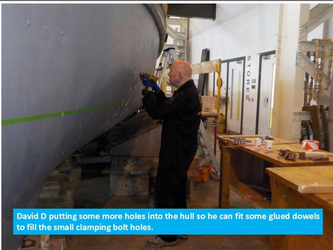
David D putting some more holes into the hull so he can fit some glued dowels to fill the small clamping bolt holes.
