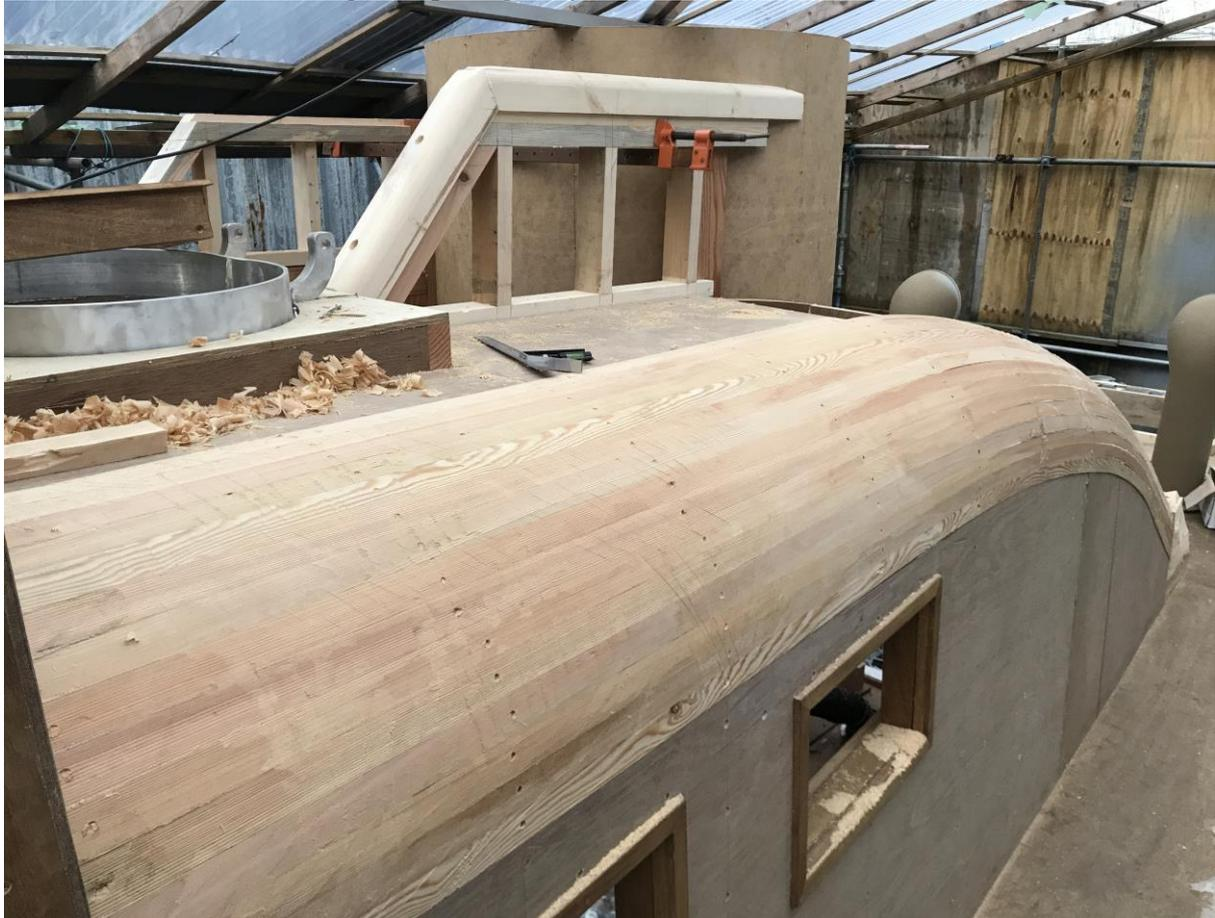
The shape is challenging as it rounds from sides to the top, and forward to aft, at the same time diminishing in width as the structure narrows towards the after deck.
