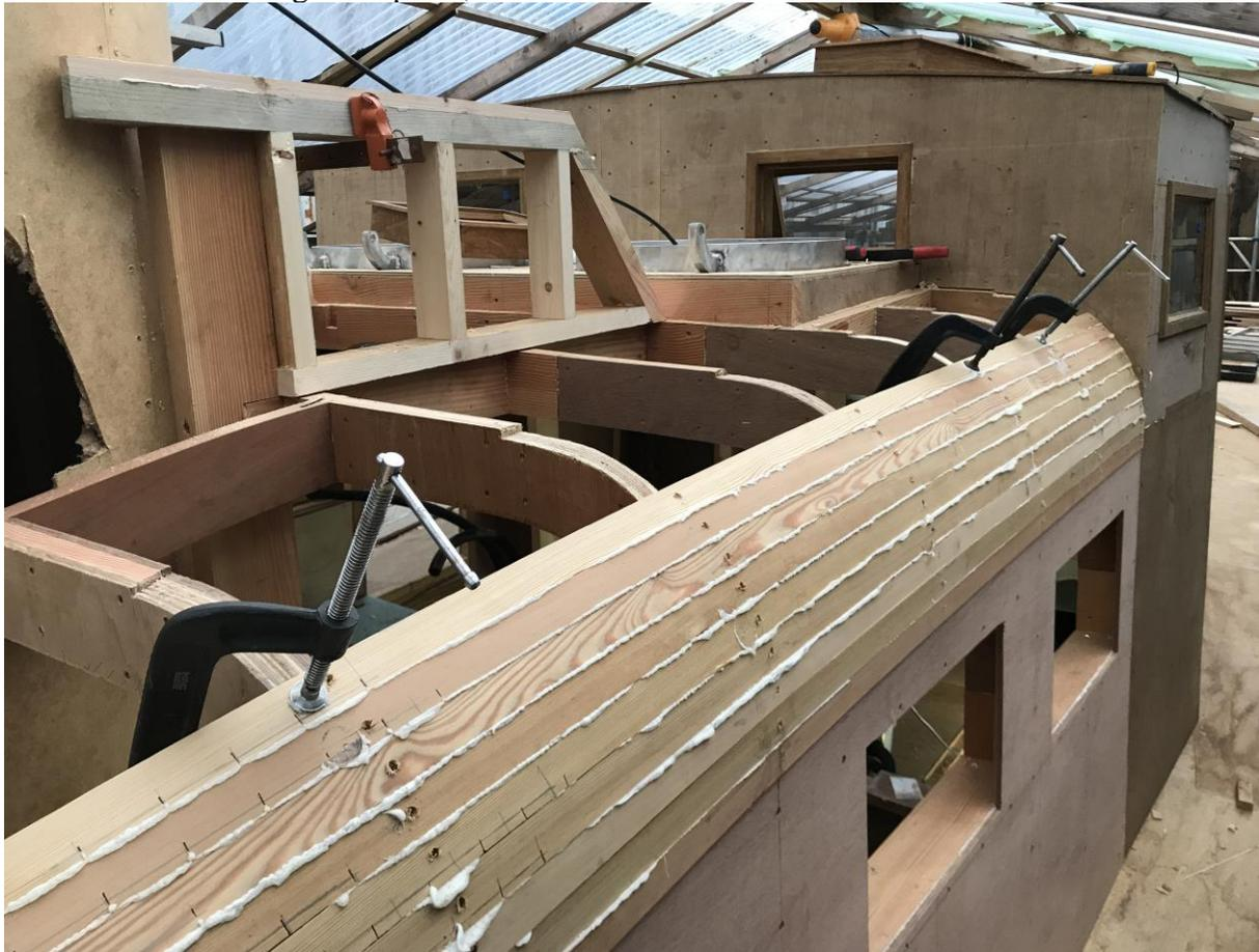
Sides have been clad in 12mm marine plywood. The rounded 'shoulders' were formed using larch battens - 14 lengths on each side, bent from the wheelhouse down to the after deck. The
